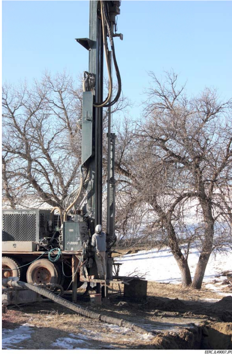
Figure 8. Groundwater-monitoring well drilling 33-12, Bell Creek, Montana (February 2013).
