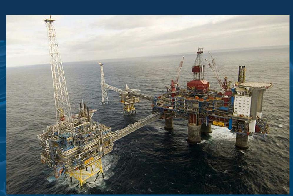
The Sleipner A CO<sub>2</sub> injection platform is on the right.<sup>3</sup>
