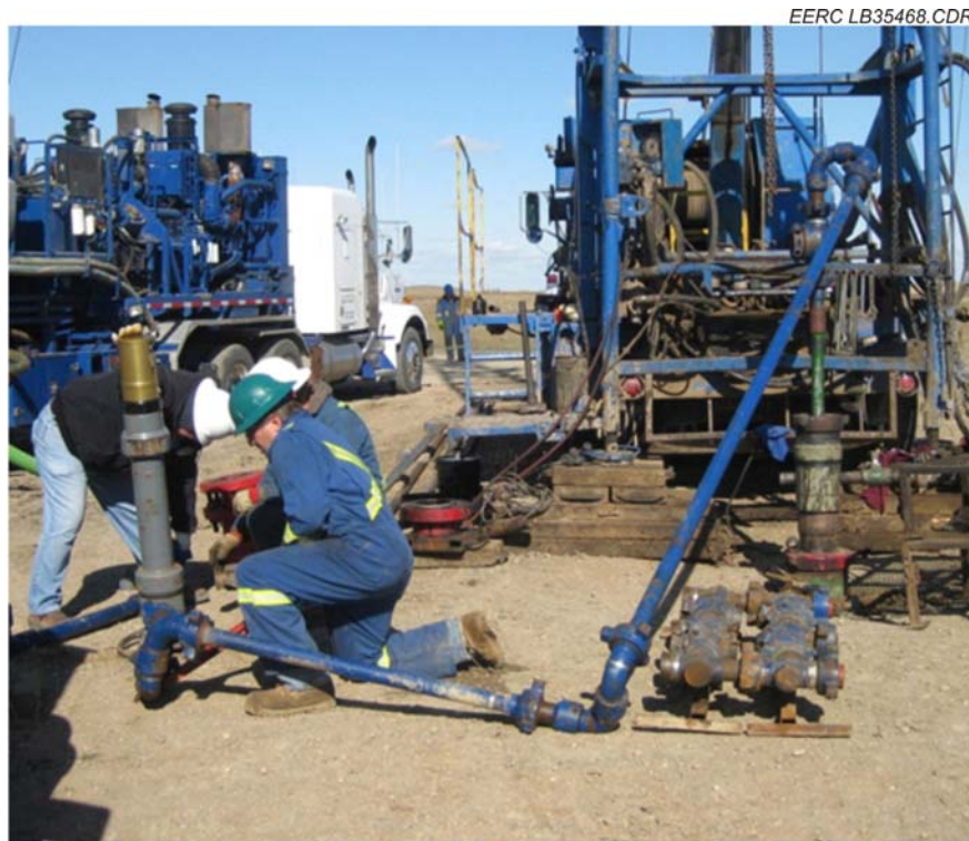
Figure 7-2. Connecting ball dropper to well for acid job.
