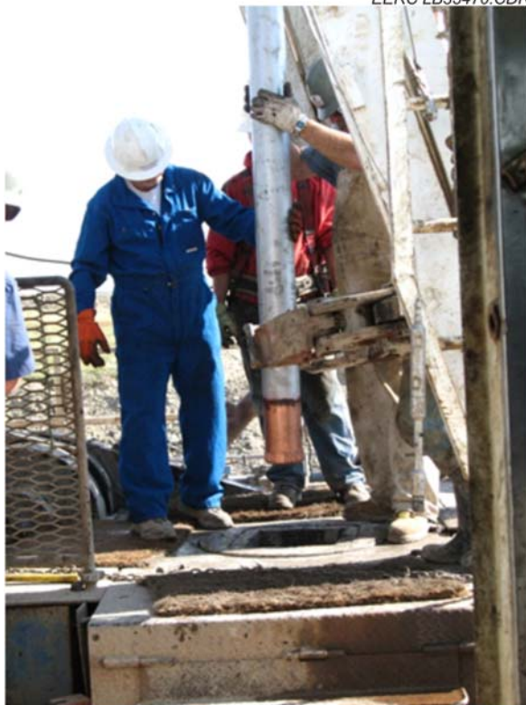
Figure 4-4. Core barrel.
