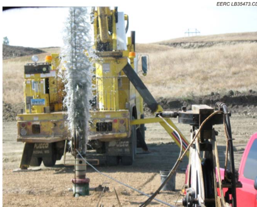
Figure 4-6. Freshwater fill leaving the borehole upon release of perforation charges.
