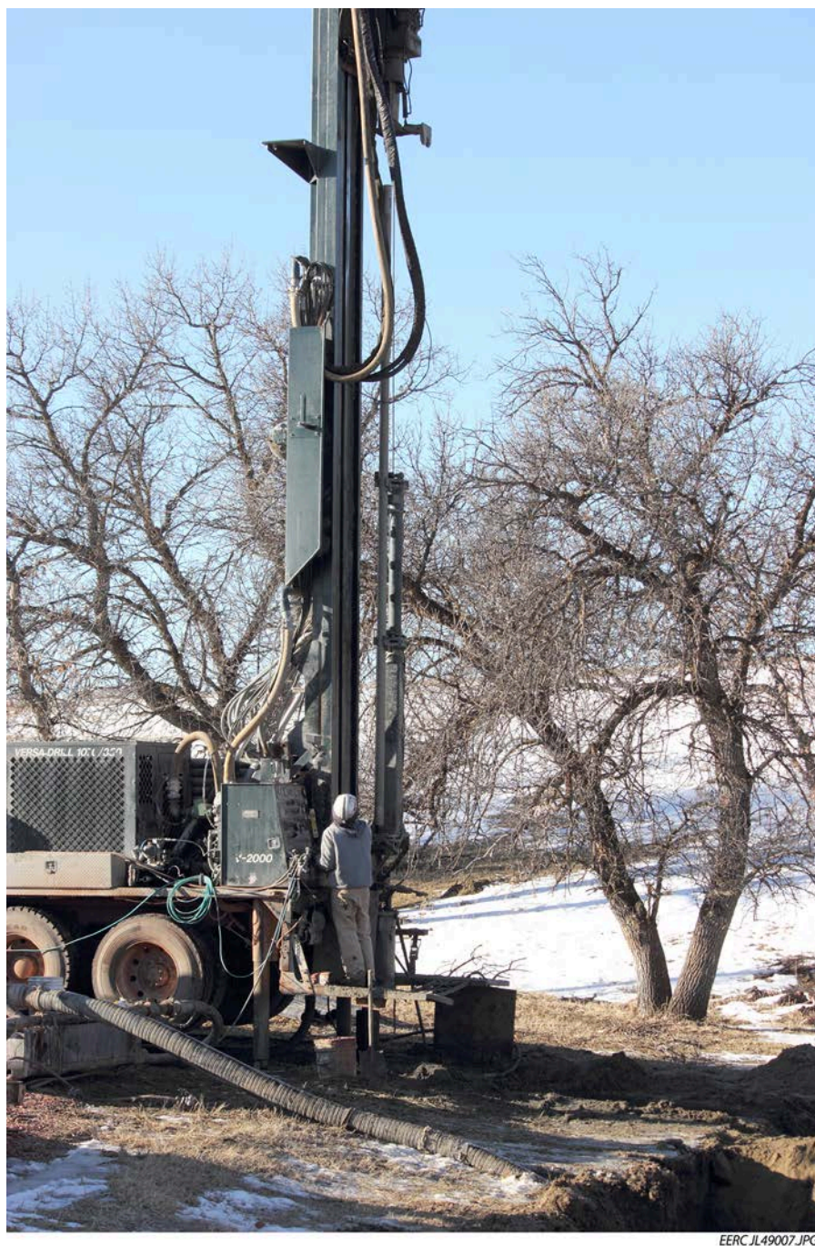
Figure 1. Groundwater-monitoring well drilling at Well Pad #3312, Bell Creek, Montana.
