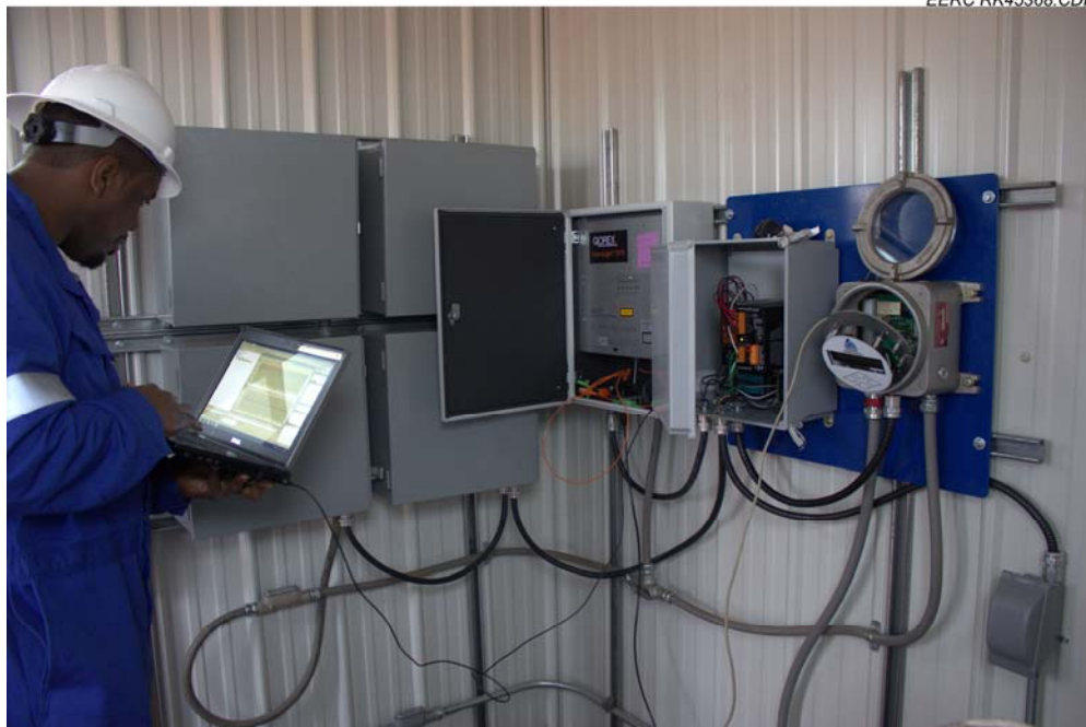
Figure 25. Qorex staff checking the functionality of the fiber optic distributed pressure/temperature data logger (leftmost open panel).
