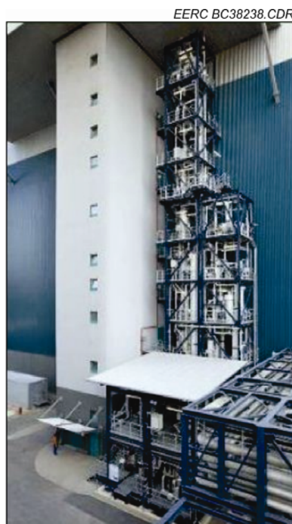
Figure 20. Postcombustion CO 2 capture pilot plant in Niederaussem, Germany (taken from Krishnamurthy and Holling, 2010).
