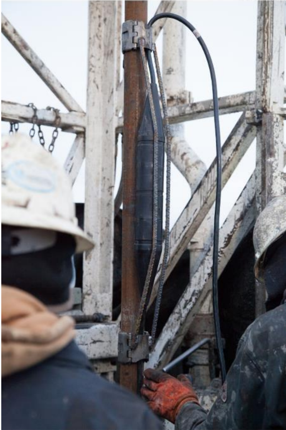
Figure 11. Each of the 50 three-component geophones was clamped to 2 \frac{7}{8} -inch tubing for installation.
