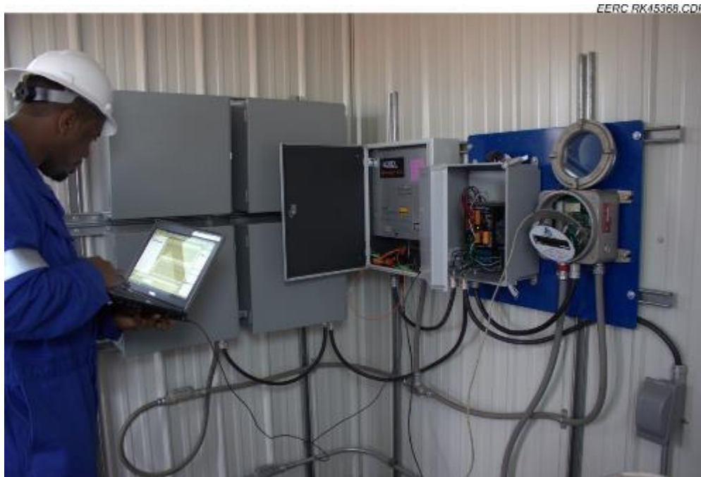
Figure 8. Qorex staff checking the functionality of the fiber optic distributed pressure/temperature data logger (left-most open panel).
