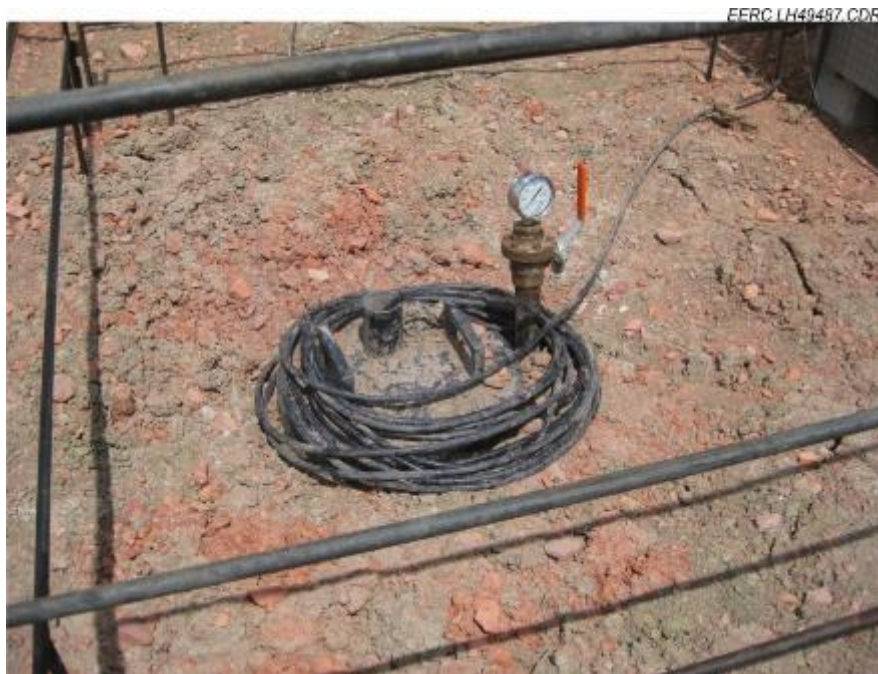
Figure 12. The 50 three-component geophones were cemented in place, effectively and permanently plugging the 04-03 OW well. The wellhead is shown here with the geophone cable coming out of the plugged well.
